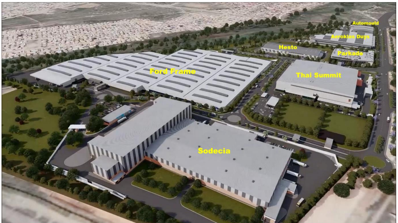
Figure 6.15 Tshwane Automotive Special Economic Zone (TASEZ) in Silverton
